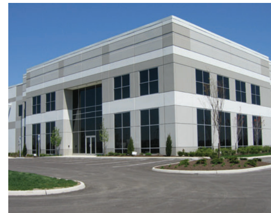
Rickenbacker Global Logistic Park's 936,000 square-foot speculative building.
